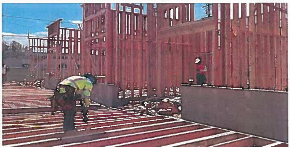
Figure 1-1. Construction of New Housing, photo by Andrew Bowen,
